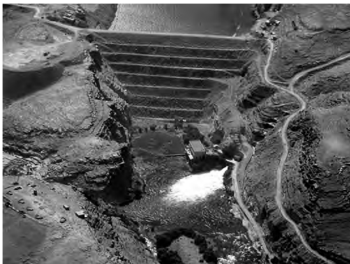
The Kajaki Dam provides flood control, power, and irrigation water to the Helmand Valley. Source: http://tiny.cc/ny92gw .
