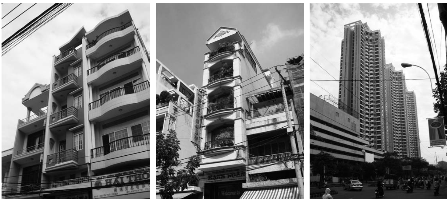
Examples of contemporary homes that are typical of new construction in the cities of Việt Nam. The first two images show four story homes above a commercial enterprise on the street level. They are known as "Tube Houses" for their narrow and deep design. The third photo is of an apartment highrise complex in Hồ Chí Minh City. Photography by Mel Schenck. You can see more of Mel's Việt Nam photos on his blog at http://layered.typepad.com/ .
