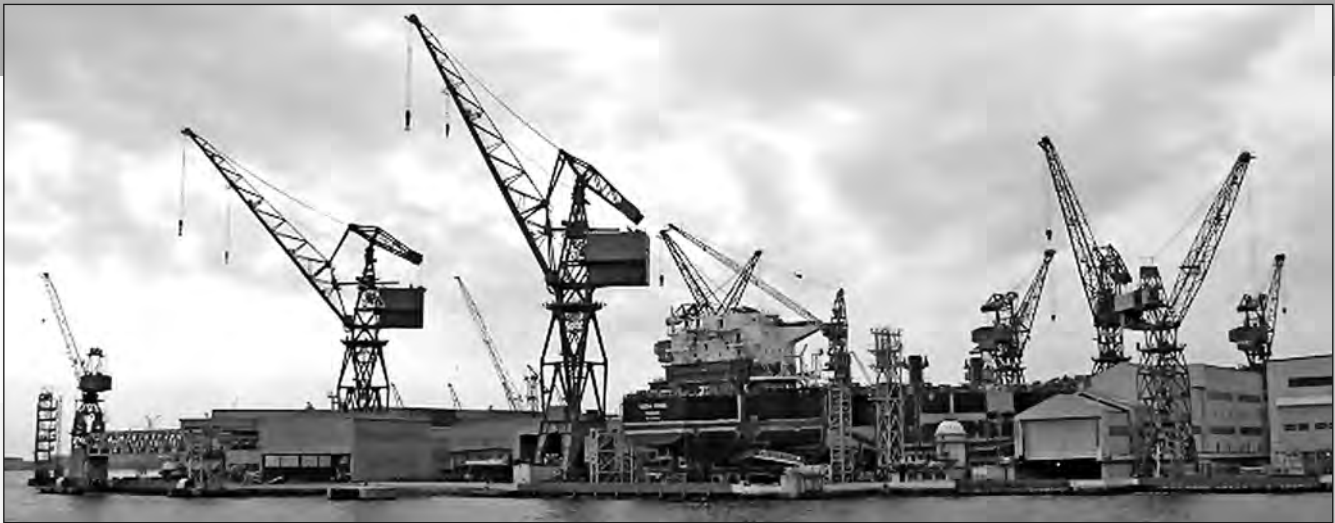
Kawasaki Shipbuilding, Kōbe Shipyard and Machinery Works of Kōbe Harbor in Kōbe, Hyōgo Prefecture, Japan. Image source: http://commons.wikimedia.org/wiki/Image:Kobe_Kawasaki_Heavy_Industries01s3200.jpg .
