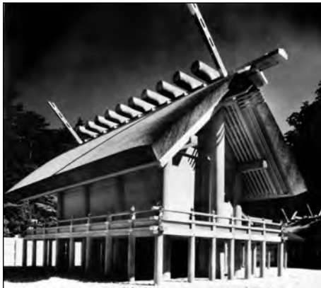
Figure 4: Main Hall of the Ise Shrine.
