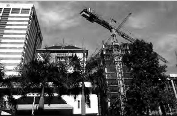
Photo 1: New construction in Jakarta. Courtesy of Christine Drake.
