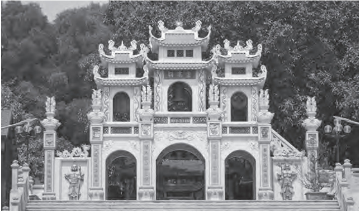
Bac Ninh, Việt Nam. The Ba Chua Kho (Queen of Stock) Temple, built during the Ly dynasty (1010–1225) on Kho Mountain, was dedicated as a national cultural historical site in 1989. Source: © Shutterstock. Photo by Yangxiang.
