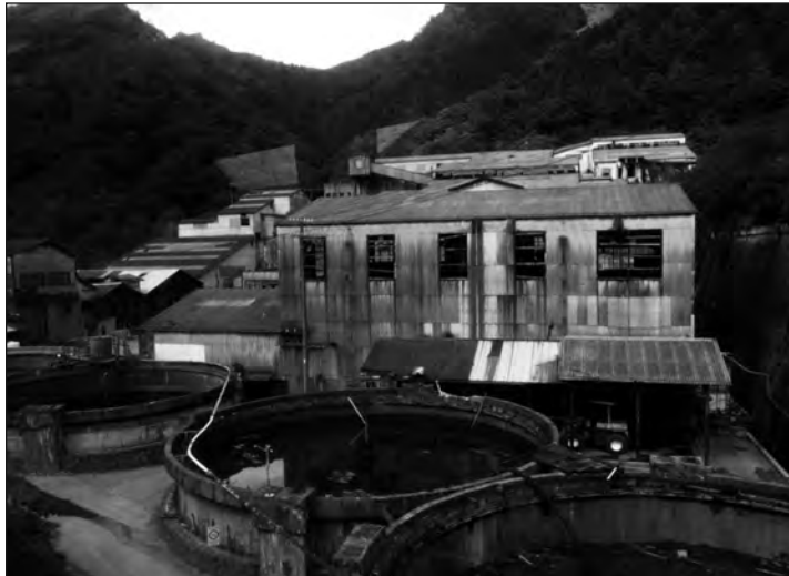
The ruins of the copper concentrating plant and sludge thickeners, Ashio Copper Mine. Photograph by Saitomo at http://www.panoramio.com/photo/14374631 .
