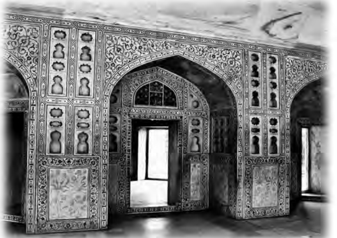
Figure 8. Decorated marble interior pointed archway in the Red Fort.
