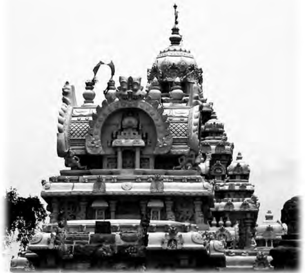
Figure 2. Façade of a Hindu Temple in South India with chattris .
