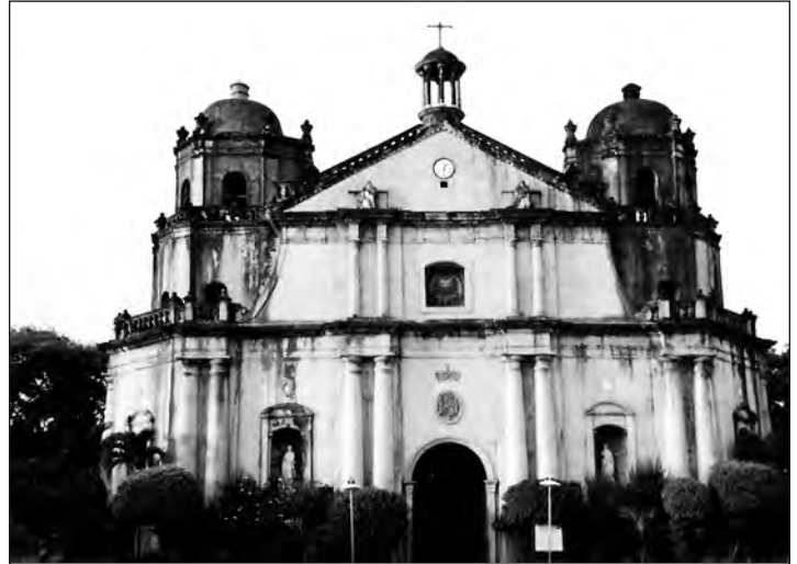
“Earthquake baroque” architecture, Naga Church, Camarines Sur.
