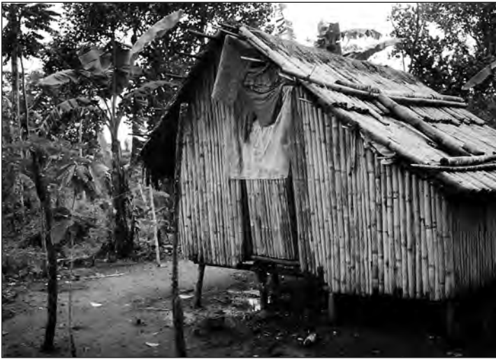
Contemporary bamboo and nipa palm house, foothills of Mt. Banahaw, Quezon Province.
