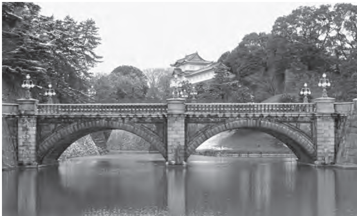
The Seimon Ishibashi bridge crosses over the moat and leads to the main gate of the Imperial Palace. Source: Wikimedia Commons at https://tinyurl.com/y2wmaoxn . Author: Kakidai.
