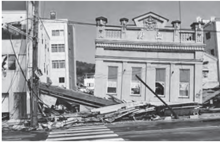
The main office building of the sake brewery in Kesennuma City was damaged by a vessel that crashed into it during the tsunami of the East Japan Earthquake.
