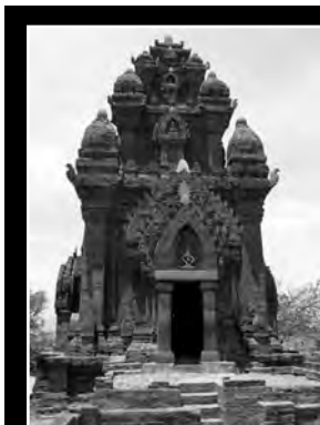
Po Klong Gerai Towers; Phan Rang, Vietnam. Photo by Mike High http://www.orientalarchitecture.com/phanrang/POKLONGGERAI02.htm
