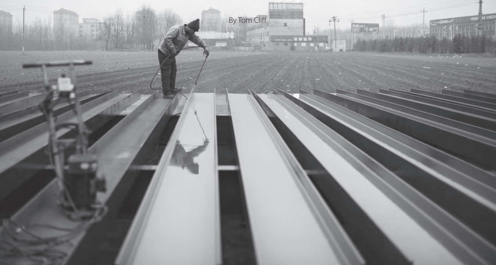
A worker spray-painting steel girders in Huagang, 2016. All photos in this article are all courtesy of the author.
