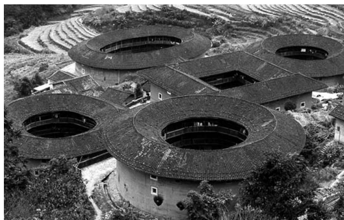
Figure 6: Some of China's most distinctive rural residences are the earthen dwellings called tulou in southeastern China. (Photo: Ronald G. Knapp)
