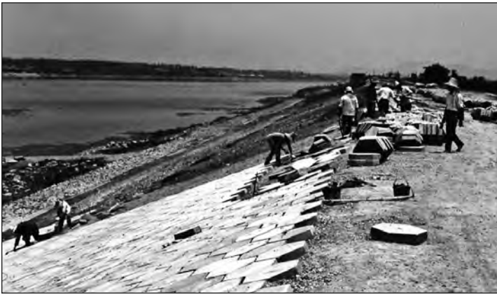
Fig. 5. Photograph of levee construction along the Fu He, a tributary of the Chang Jiang.
