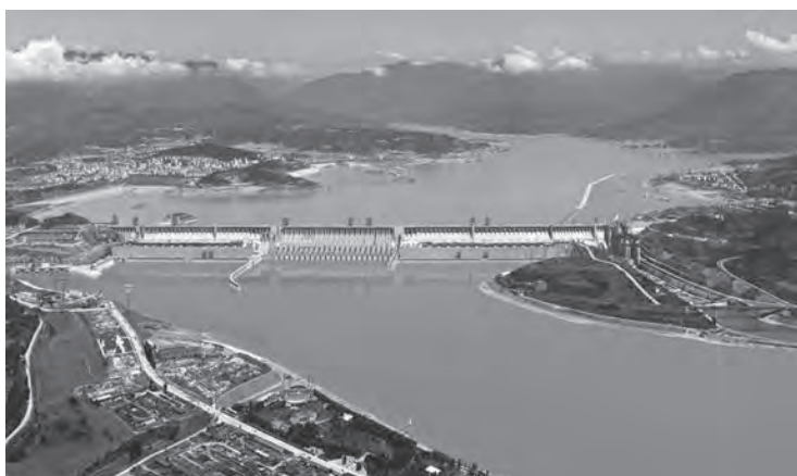
Aerial view of the Three Gorges Dam—the world's largest hydropower plant. Source: IFS website at https://tinyurl.com/y9w9bdky .
