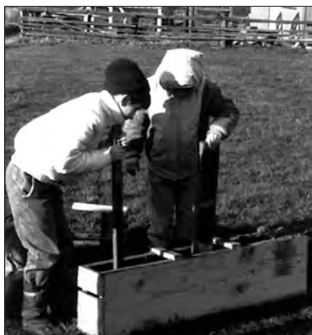
Students tamping dirt in the forms to make a section of the wall.
