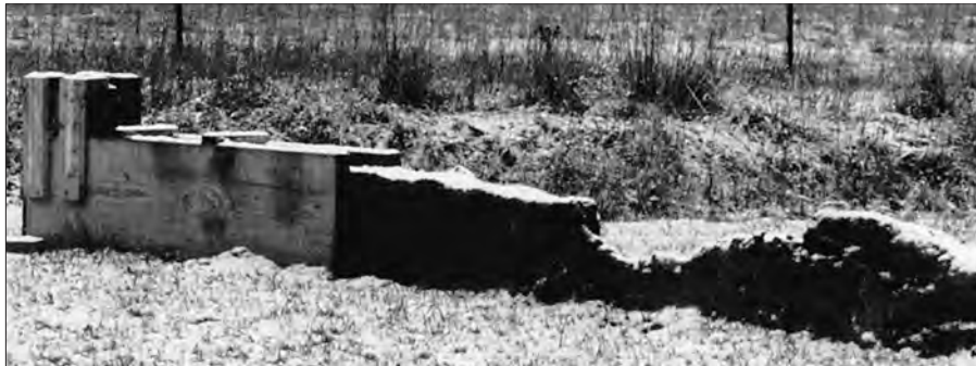
"Wall" forms at left, partly constructed sections in center, collapsed sections.
