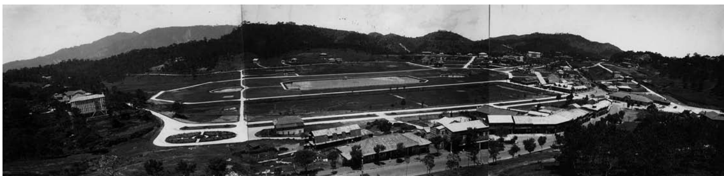
Figure 6. A view of the core of Baguio in 1926 (Rizal Library, Ateneo de Manila University). 15
