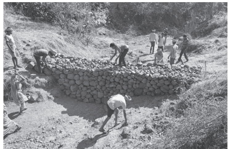
Stone gully plugging in Sagai Village as part of watershed development. Source: Photo by Trupti Mehta.
